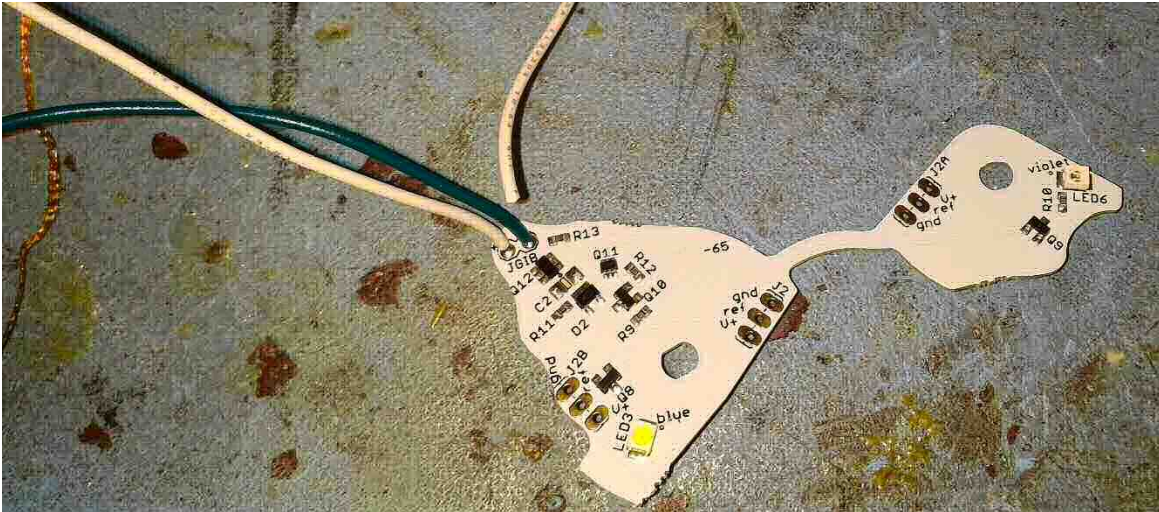
Figure 4 Solder GI wires to JGI and JGIB
