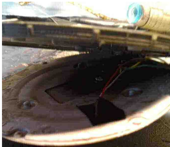
Figure 10. Secure loose VCC & SW
